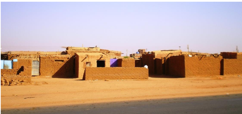
Photo No. 5: Informal Housing, Omdurman Photo by Gamal M. Hamid
