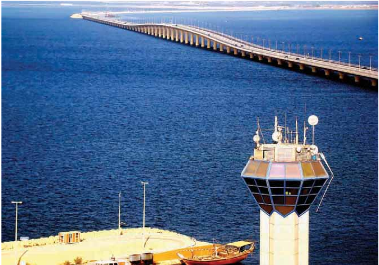
☒ The 25 km King Fahd Causeway linking Saudi Arabia to Bahrain. ©Mohamed Ghuloom. Licensed under the Creative Commons Attribution 3.0 Unported license.
