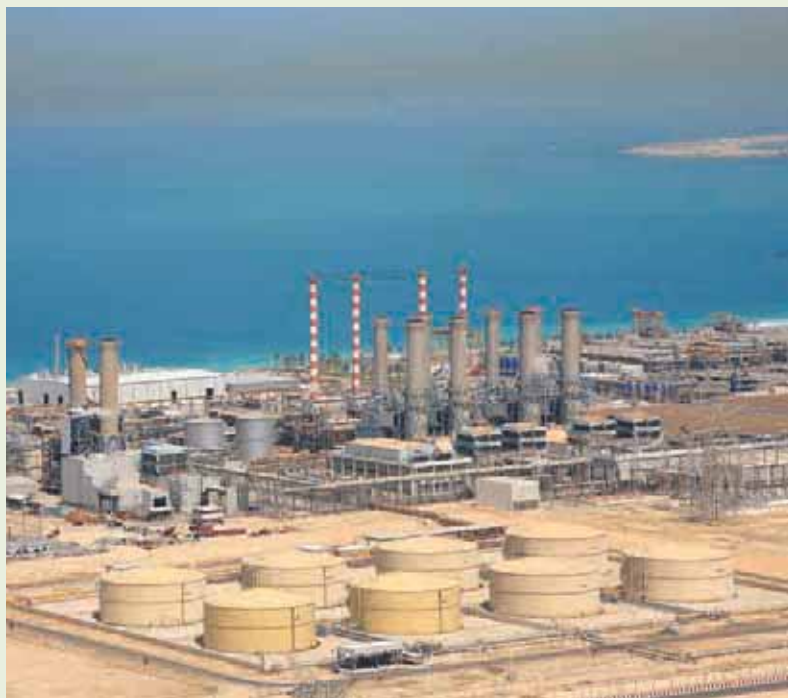
Desalination plant in Dubai, UAE. ©Shao Weiwei/Shutterstock
