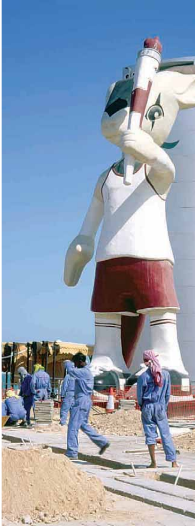
☒ Doha, Qatar. Asian labourers at work on the drainage system in front of Qatar's national "Orry the Oryx" mascot, originally created for the 2006 Asian Games. Qatar's impressive infrastructure is being created by a vast army of cheap labourers drawn from across Asia. ©Paul Cowan/iStockphoto
