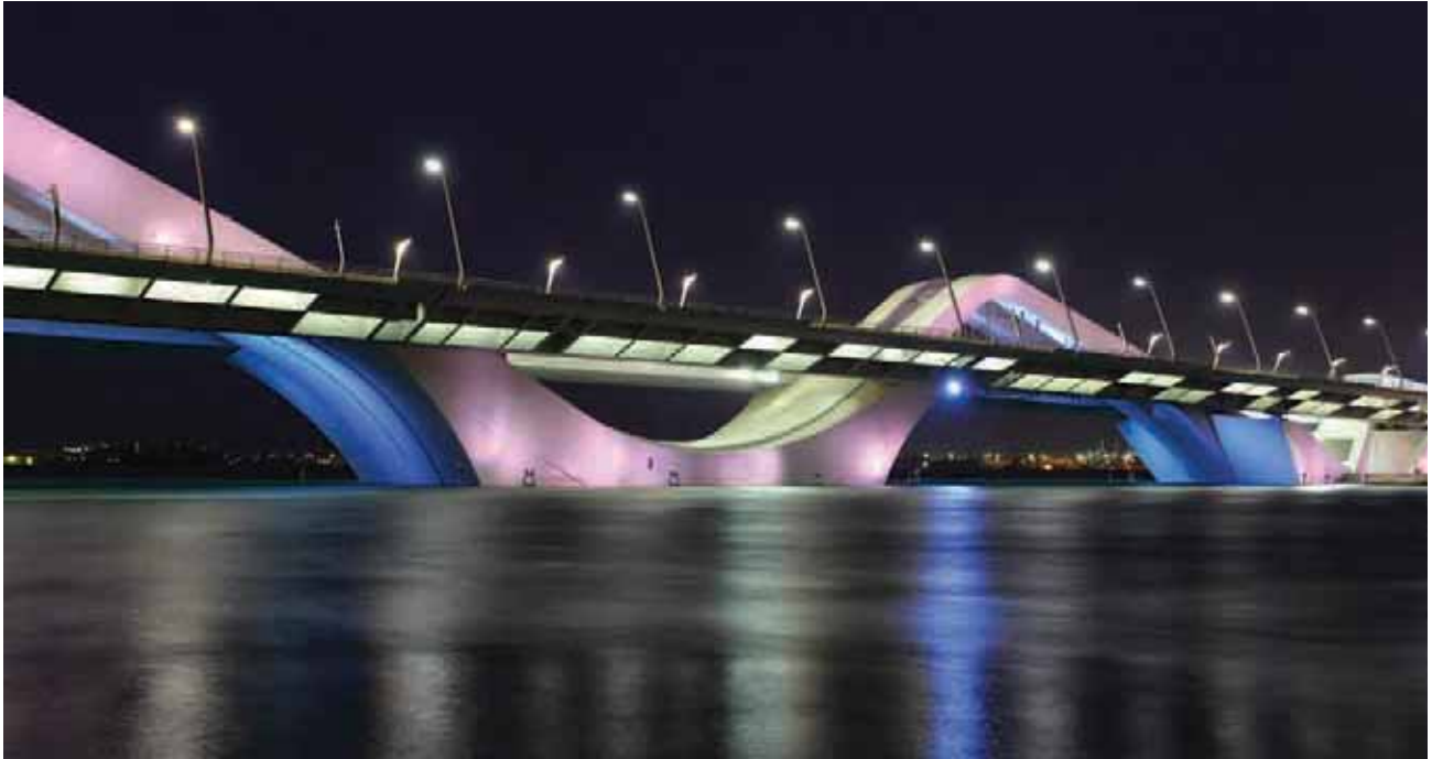
Opened in November 2010, the 842-meter-long Sheikh Zayed bridge in Abu Dhabi is said to be the most intricate bridge ever constructed. ©Philip Lange/iStockphoto
