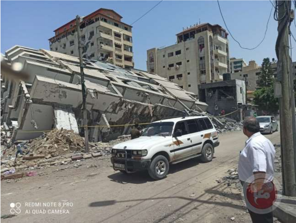
Figure 20: Destroyed Palestinian houses during the Gaza war 2021. Source: Ma'am Agency (2021).
