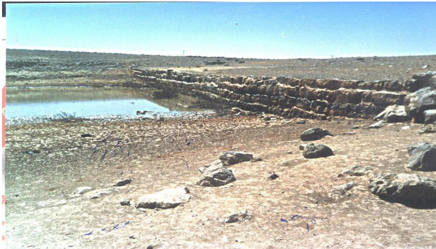
Figure 9.4: Small earth dam, an indigenous practice for water harvesting in dry region
