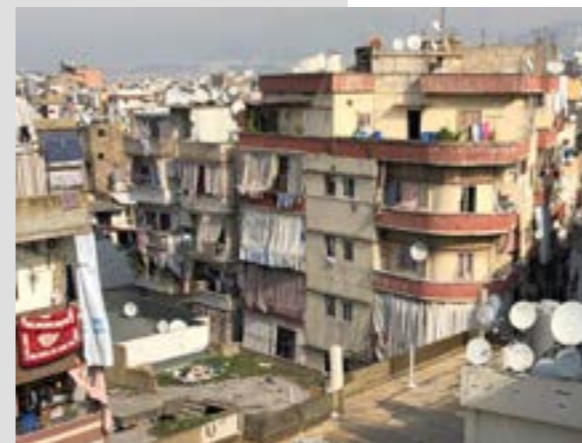
Damaged buildings in building in Naba'a, Lebanon (UN-Habitat, 2021)
