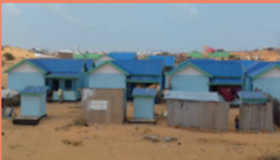
Photo 18: New homes in Kismayo / UN-Habitat
