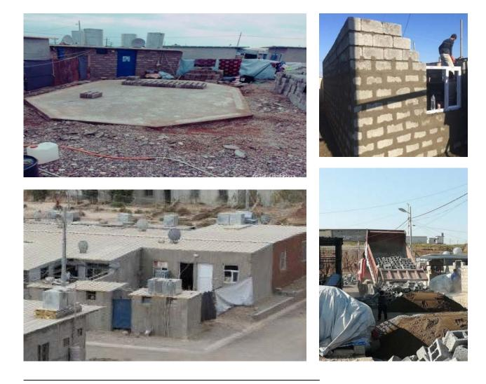
Figure XXIII: The upgraded shelter in implantation by PWJ. The images show the process of provision and self-built. Source: PWJ, 2019.
